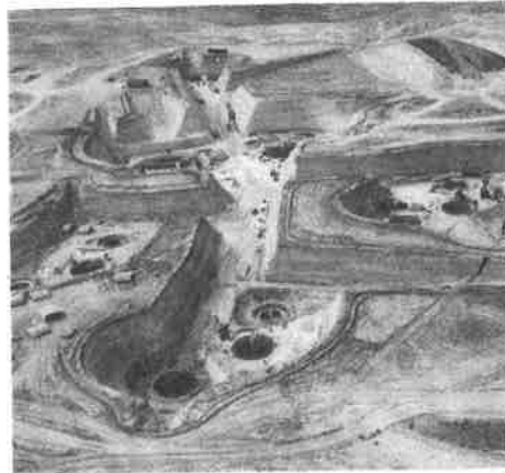
Construction of Launch Sites Titan ICBM, Lowry AFB
