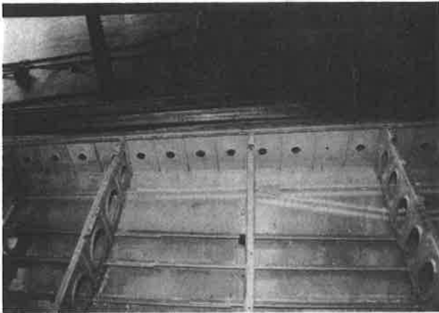
OPEN WING SECTION (Corrosion removed, etched, alodized, & painted)
