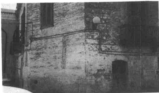
6.) Same Villa - Another View
