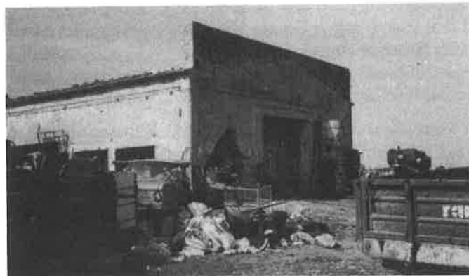
10.) Same Building (This end was set apart for EM Shower Room)
